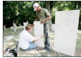
Helen Wildermuth and Raul Martinez of Stonehugger Cemetery Restoration of Indiana use epoxy to put together one of the broken headstones in the Harrington Cemetery in Harris Township just west of Elmore. (THE BLADE/DAVE ZAPOTOSKY)
